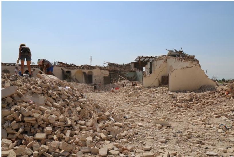
Remnants of Villa Fini (F4, collapsed weak brick structure) in western Mira (photo: Alberto Gobbi)
