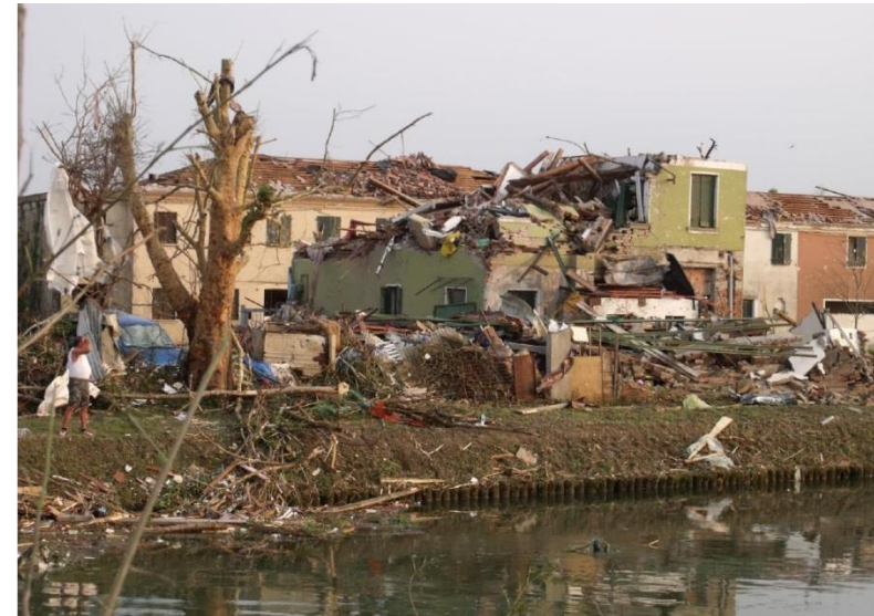
F4 damage (strong brick structure, walls partly collapsed) in western Mira close to the Villa Fini, on the other side of the streamer (photo: Alberto Gobbi)
